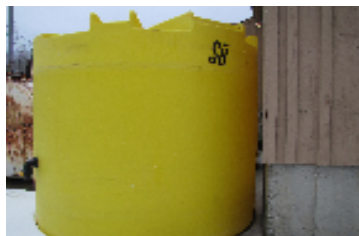
3,000 Gallon Salt Treatment tank
